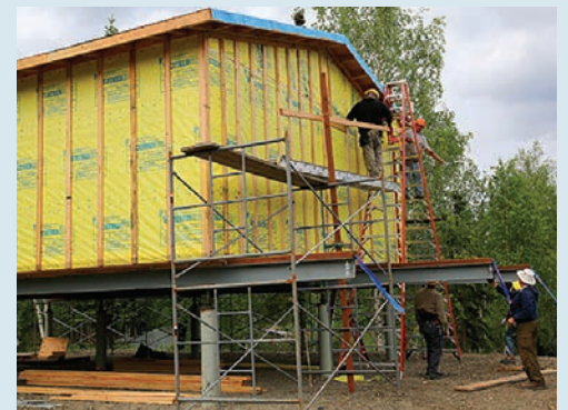
Galena, Alaska, where Yukon River flooding destroyed 90% of the buildings in 2013. Photo by Eliza Hotchkiss, NREL, 32755
