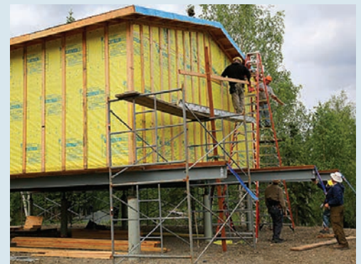
Galena, Alaska, where Yukon River flooding destroyed 90% of the buildings in 2013. Photo by Eliza Hotchkiss, NREL, 32755
