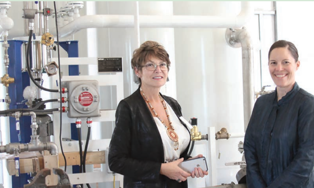
Blue Lake Rancheria Vice Chairperson Arla Ramsey and Energy Director Jana Ganion survey the progress of the Tribe's biomass-to-fuel cell power plant, scheduled to go online this spring. Photo from Jana Ganion, Blue Lake Rancheria, NREL 32766
